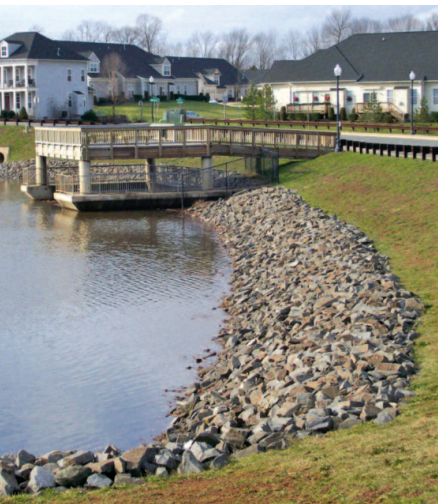
Stormwater Retention Pond, Manassas, VA. Photo by Manassas Dept. of Community Development
